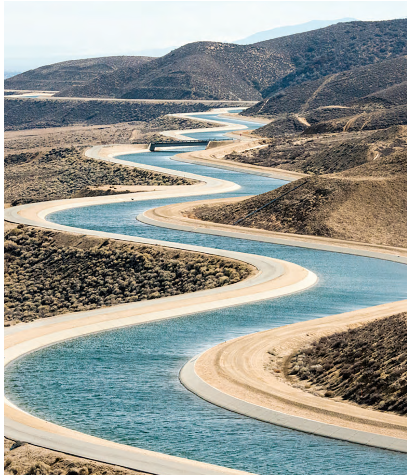
The State Water Project canal, a major conduit for imported water for the Basin.
